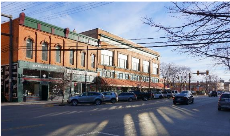
Figure 4: Historic businesses like the Duhamel Building on Sixth Street have been part of the Downtown Historic District since the 1970s.
