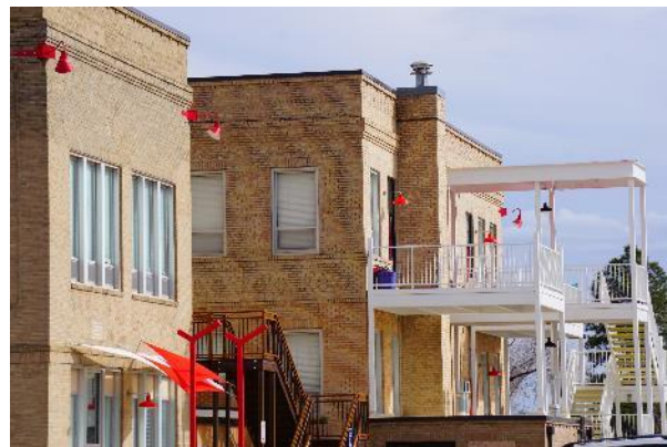
Figure 14: The conversion of James A. Garfield Elementary School into modern, residential apartments is an example of successful adaptive reuse.
