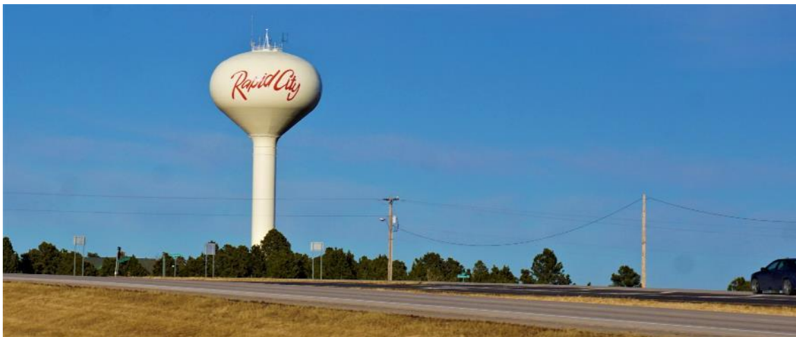
Figure 25: Historic preservation planning can help Rapid City prepare for growth.
