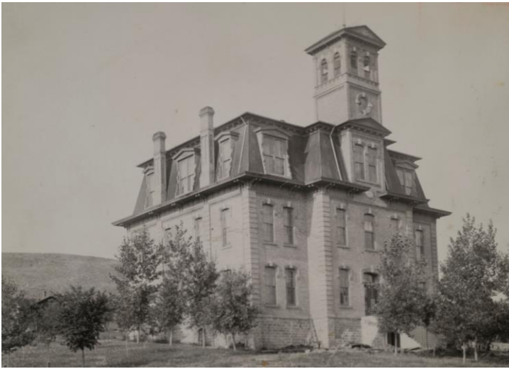
“First Rapid City High School, cost $12,000, south side of Columbus between 6 th and 7 th ” Minnilusa Historical Association
