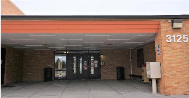
Meadowbrook Elementary School
