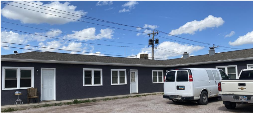
Former Model Motel – North Maple Street.
