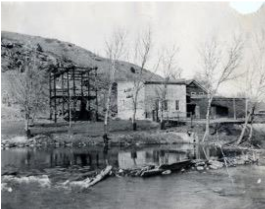
Sub-Station at base of Cowboy Hill Minnilusa Historical Association
