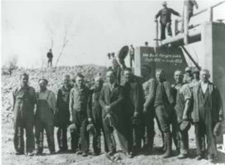
Construction of the Canyon Lake Dam, 1933 Minnilusa Historical Association
